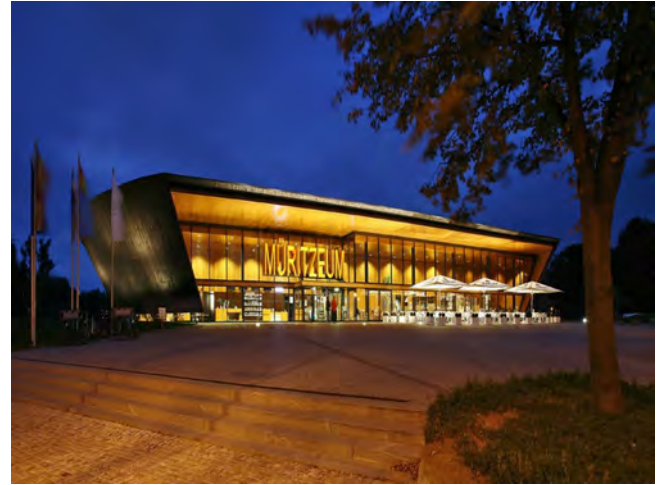
Figure 2. The new exhibition building “House of 1000 Lakes” (Photo: Mirko Runge).
