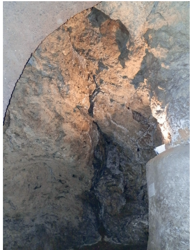
Fig. 23: Svatý Jan pod Skalou, cave accessible from the monastery. Paleozoic limestone (right) and Holocene travertine (left) (photo: L. ZÖLLER).
